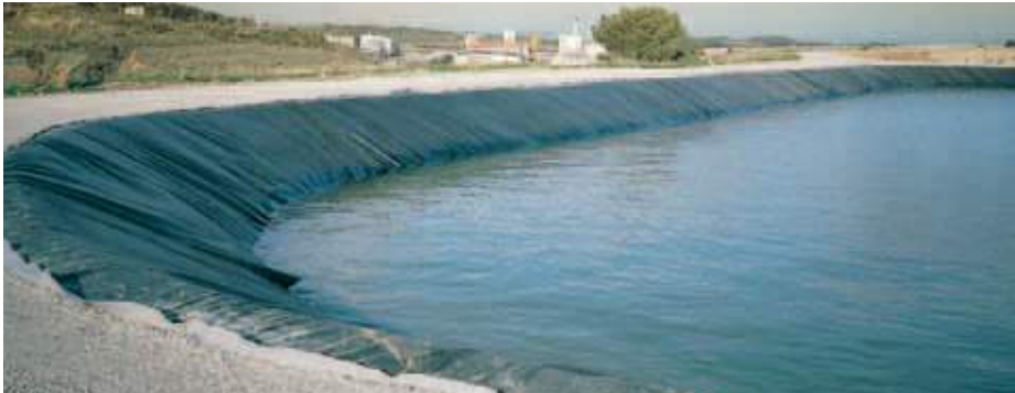
80000 m² Waste water reservoir, Comurhex, Norbonne, France.
