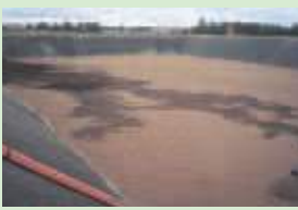
2001 AvestaPolarit, Avesta, Sweden Liner in industrial landfill for hydroxide sludge. 7.100 m²
