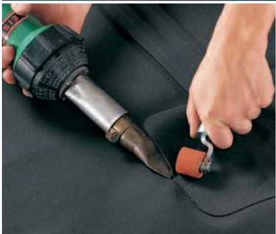
Prefabricated pipe boots, flashings and details are seamed with hot air guns. Quality control testing is provided by means of high pressure air lance testing.
